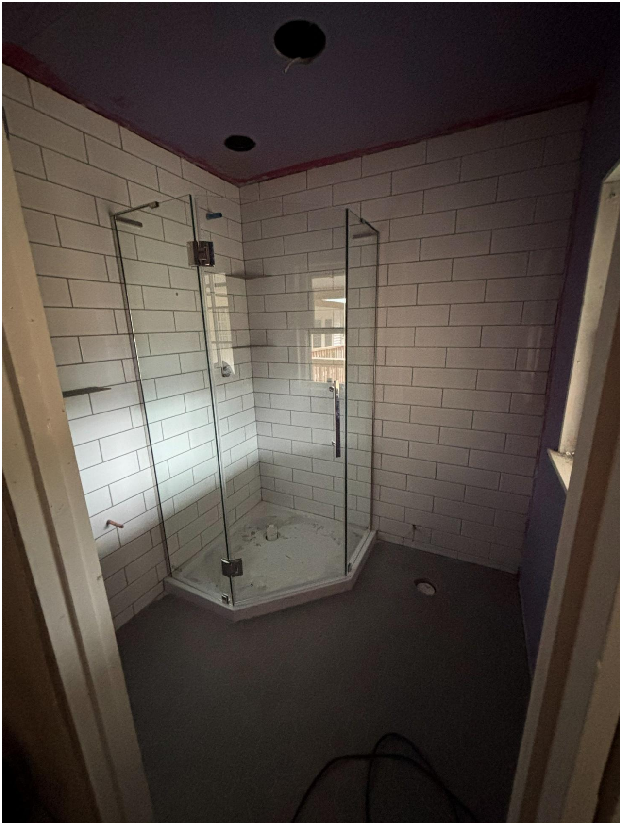
A sneak peek at Room 12's new bathroom:
